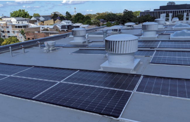
TPO Membrane Australia | 325kW
