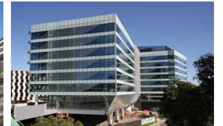
MELBOURNE WATER AUTHORITY Melbourne, Australia 6 Star Green Star certificate
