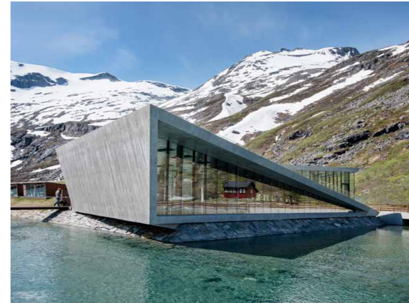
TROLLSTIGEN MOUNTAIN PASS PUBLIC TOILET Rauma, Norway
