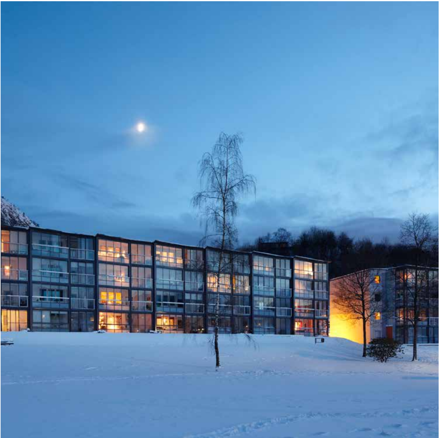
Integrated solar panels, laminated in glass. Here, the glass in the cladding is used to generate energy.
