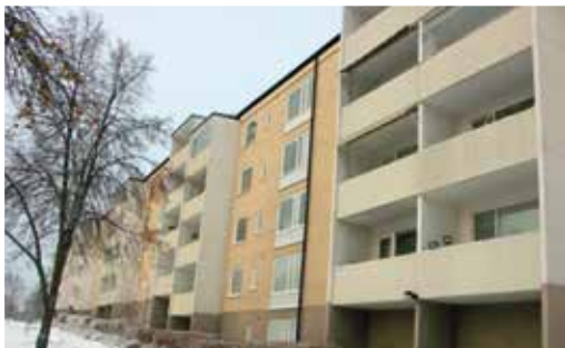
Traditional renovation of open balconies is expensive and time consuming and must be repeated about every 15 years.
